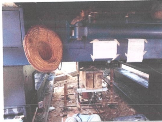
Photo 3.17 Hydraulic Jack-In Pile Machine
