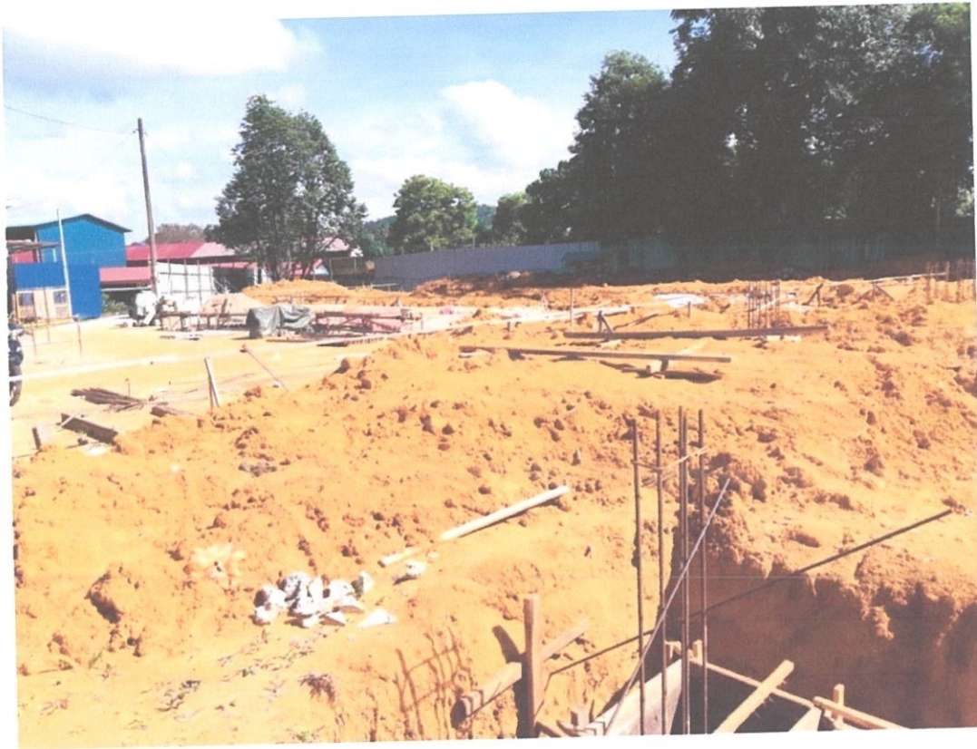
Photo 3.27 Site Condition View
