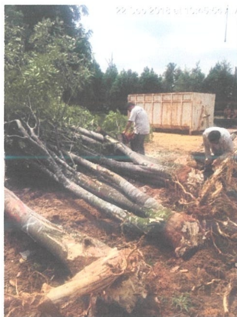
Photo 3.11 Tree cut into pieces using the chainsaw
