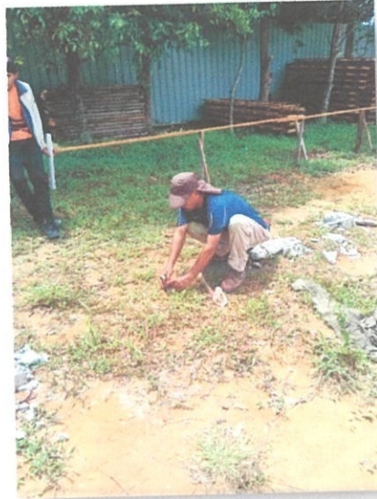
Photo 3.25 Putting the prismatic level to the centre of the point load
