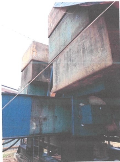
Photo 3.16 Cubical Load as weight for the hydraulic piling machine.
