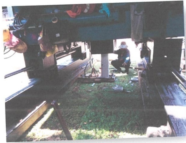
Photo 3.21 Positioning of piling bars.
