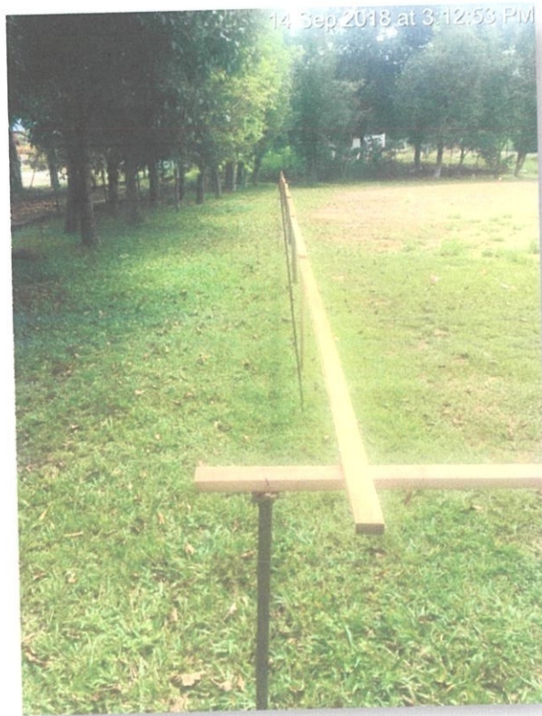
Photo 3.6 Offset peg being pegging in to marks the site area.
