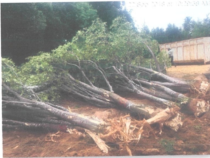
Photo 3.8 Demolition process of cutting off all this tree.
