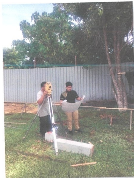
Photo 3.26 Measurement will be recorded to an As-Build drawing.
