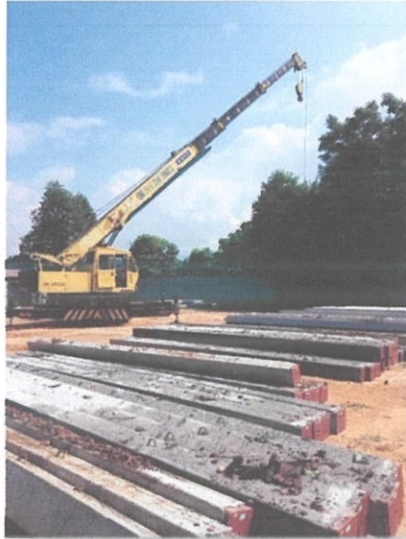
Photo 3.19 Crane is used to rearrange all the piling bars.
