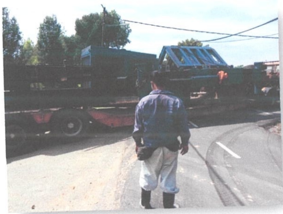
Photo 3.13 Brought in the piling machine.
