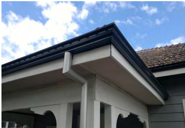
Figure 1 : The Gutter and Rainwater Downpipe
