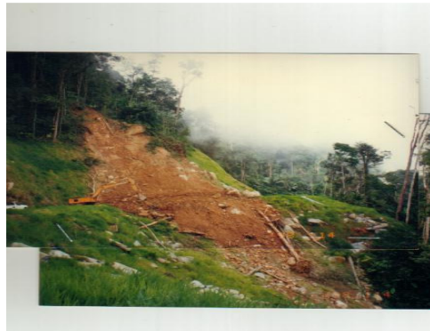
Fig. 5 : The typical slope failure along Jalan Baru Gap to Fraser Hill
