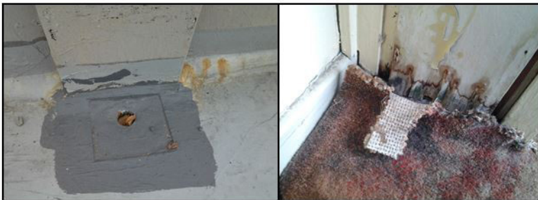
Figure 3: Roof and RWDP Failure Cause Timber Column Damage, Moisture and Mould Growth at Library
